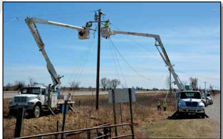
CEC linemen string and pull new wire on a section of our system south of Osceola and just west of I-35 near the County Road H45 exit. The heavier wire is part of a larger project to complete a three-phase tie line between the Hopeville, Osceola and I-35 substations. This will improve system reliability and provide redundancy on our system in order to backfeed power between substations.
