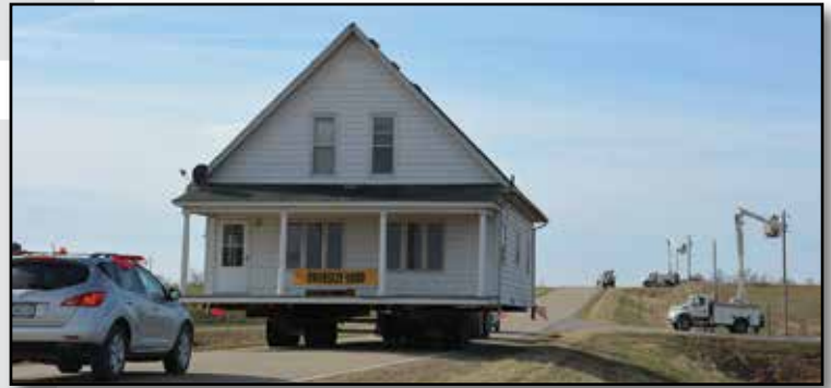
CEC linemen stay ahead of a house move, removing overhead lines as the house passes through our service territory to its destination south of Allerton.
