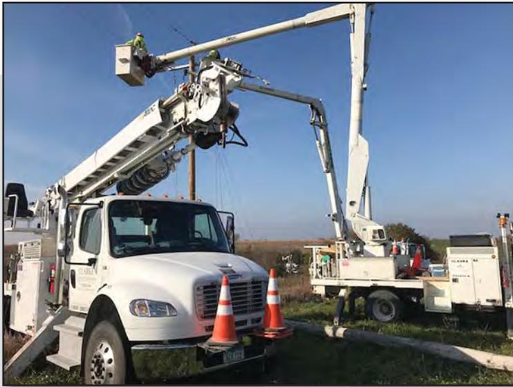
**CLARKE ELECTRIC CREWS** finished working in the Williamson area making a system improvement to alleviate failing underground infrastructure. The three miles of line were identified as a problem area in the cooperative's construction work plan during our annual planning. Our field staking engineer begins the work by assessing the area to determine the most efficient route to locate the poles and lines while balancing the load the lines will carry to the end user, you, our member.
